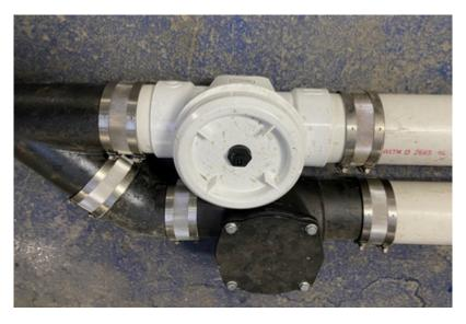
Backflow valves are specifically designed to block the drainpipes temporarily.
